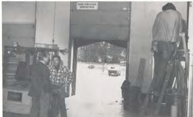
Austin Bassett, consulting engineer (left), discusses alterations to the Annacis plant with ZERO-LOCK employees Jim Walden (centre) and Ken Evano. The pair were dismantling the prefabricated wall, built by their company, between the finished storage room and the product room.
