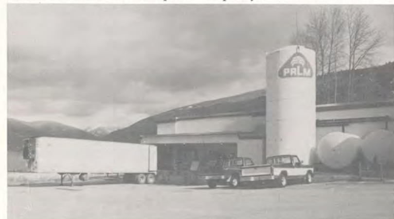
The Nelson facility was built in 1967 as a sister plant to the one in Prince George.
