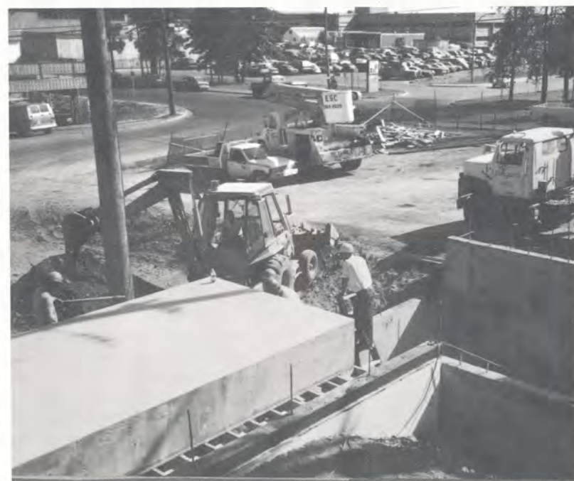
In Prince George, construction employees build foundation for ice builder, which is used during production in the day and to make ice at night.
