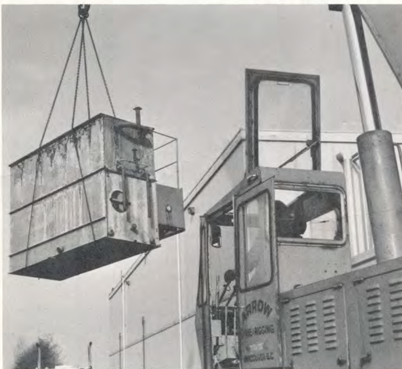
Out with the old condenser...
