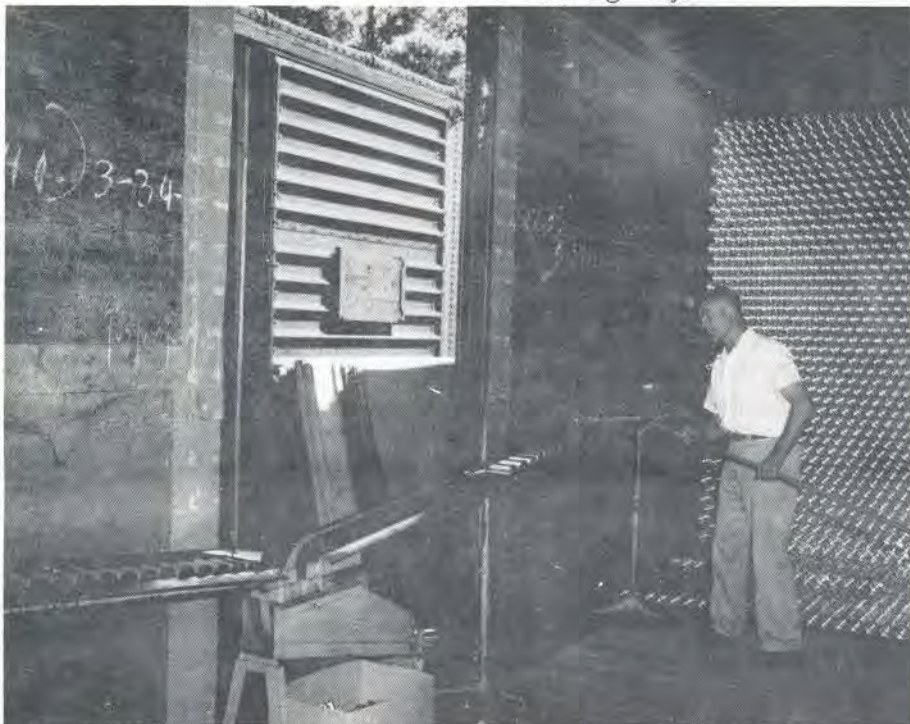
This photo was taken 20 years ago at the unloading area of the Pacific Milk plant. It shows how tins were unloaded: by hand, 18 at a time. Today the unloading operation is more mechanized and the "rake" this employee is using is part of history.
