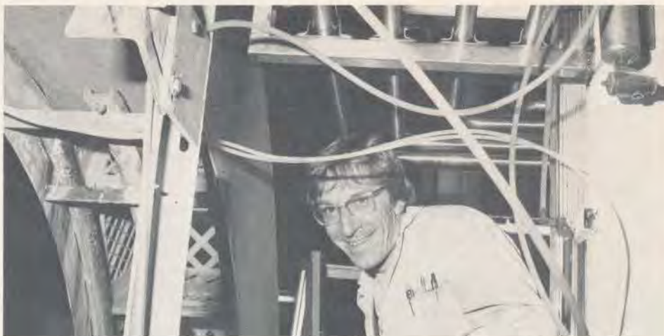
The piping above Al Wheatley will provide cleaning water to all fluid-line machines.
