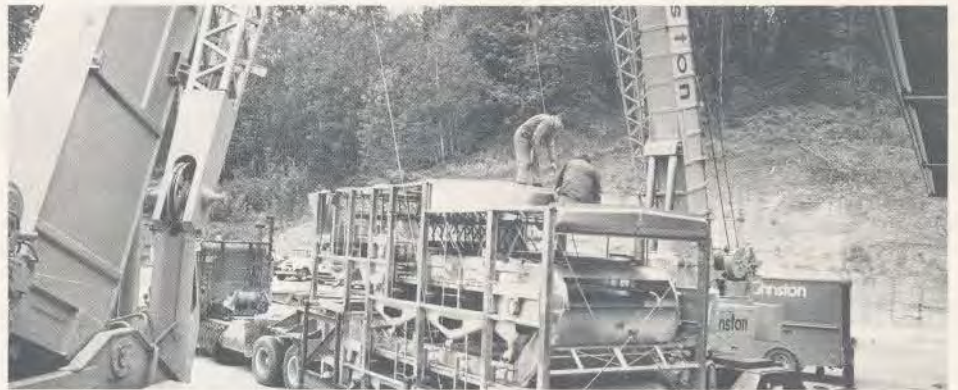
Bottom part of Little Alfie cheesemaking equipment is moved from truck to plant dock.
