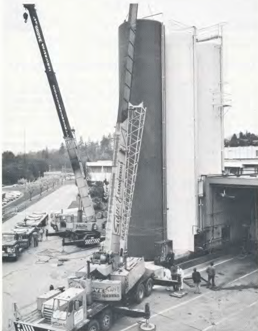
A third refrigerated silo tank has been installed on a preconstructed foundation at the Burnaby Plant. This completes facilities which were planned several years ago to allow more raw milk to be stored over a shorter work week and holiday weekends. This 428,000 capacity silo came from Wisconsin by train and was unloaded at Lake City.
