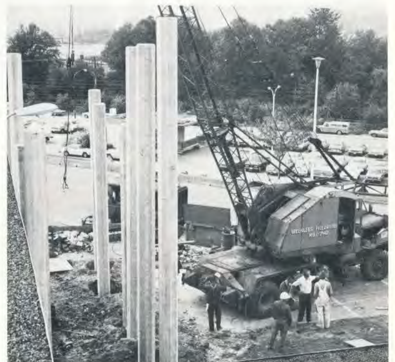
A continual thumping was heard for several days at Burnaby when twelve pre-cast concrete piles were driven outside the plant. They form the basis of support for a four-foot thick concrete platform which is the first step in a planned expansion of the production area. The platform, which will eventually hold three new raw milk tanks, weighs 400,000 pounds and contains 100 yards of concrete. The supporting piles were necessary since the soil in that area contains a three-foot layer of peat which would allow settlement. Holes were first drilled about twenty feet below ground level and the piles were driven down six feet deeper.
