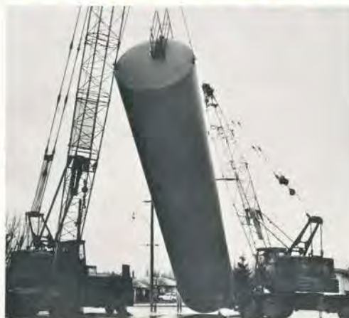
TRICKY JOB of upending tank is accomplished with two cranes which work together to place the tank on previously constructed concrete foundation. Job Foreman rides down on lifting boom after unhooking steel hoisting cables. The tank stands about 70 feet high on its foundation and can be seen from the freeway on a clear day.
