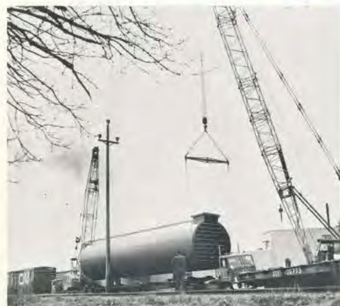
SILLO STORAGE TANK arrives at Sardis Plant on rail car. It is lifted by two cranes onto low bed truck for hauling to tank foundation. The 200 ton capacity tank will be used for receiving and storing raw milk. The inner shell of the tank is stainless steel; the outer shell is mild steel coated with an epoxy resin, with a three inch insulation in between.
