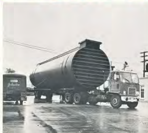
SILLO STORAGE TANK arrives at Sardis Plant on rail car. It is lifted by two cranes onto low bed truck for hauling to tank foundation. The 200 ton capacity tank will be used for receiving and storing raw milk. The inner shell of the tank is stainless steel; the outer shell is mild steel coated with an epoxy resin, with a three inch insulation in between.
