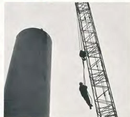
TRICKY JOB of upending tank is accomplished with two cranes which work together to place the tank on previously constructed concrete foundation. Job Foreman rides down on lifting boom after unhooking steel hoisting cables. The tank stands about 70 feet high on its foundation and can be seen from the freeway on a clear day.
