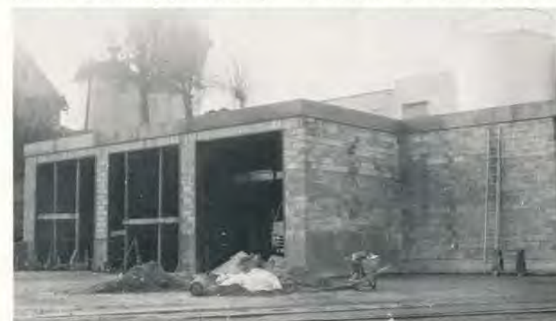
BECAUSE OF THE INCREASED volume of milk that the Delair Plant will handle with the termination of can milk shipments, a 100,000 pound silo tank was installed. In addition to this three new truck bays are being built to provide protection for the farm tankers while they are at the plant.
