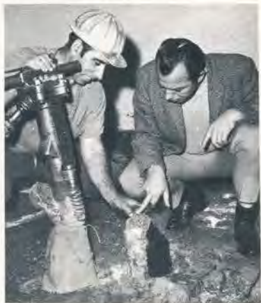
TONY CABRAL of Allan and Viner construction, with JACK SLYKERMAN of the Sardis engineering department look at the old concrete floor in the can dump room. What should have been an easy day's work stretched into several as the construction crew found that the floor, poured in the 1920s, was meant to last.
