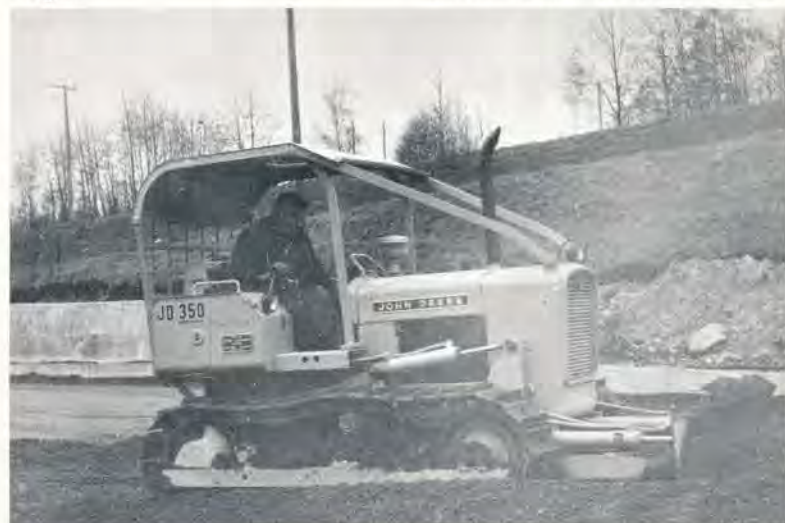
INCREASED TRAFFIC around the wholesale dock at the Burnaby Plant has forced the widening of the roadway. The cat is levelling gravel making it ready for blacktop.
