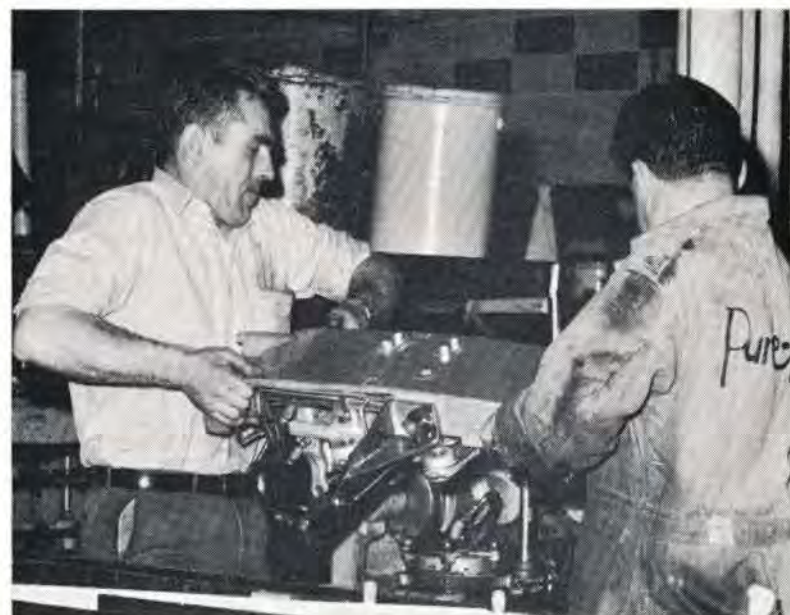
The new rear bridge on a Pure-Pak machine is hoisted into place, above, by two of the mechanics who installed the equipment here. Many adjustments and changes had to be made in the Burnaby plant's fluid production line during the switch-over this spring.
