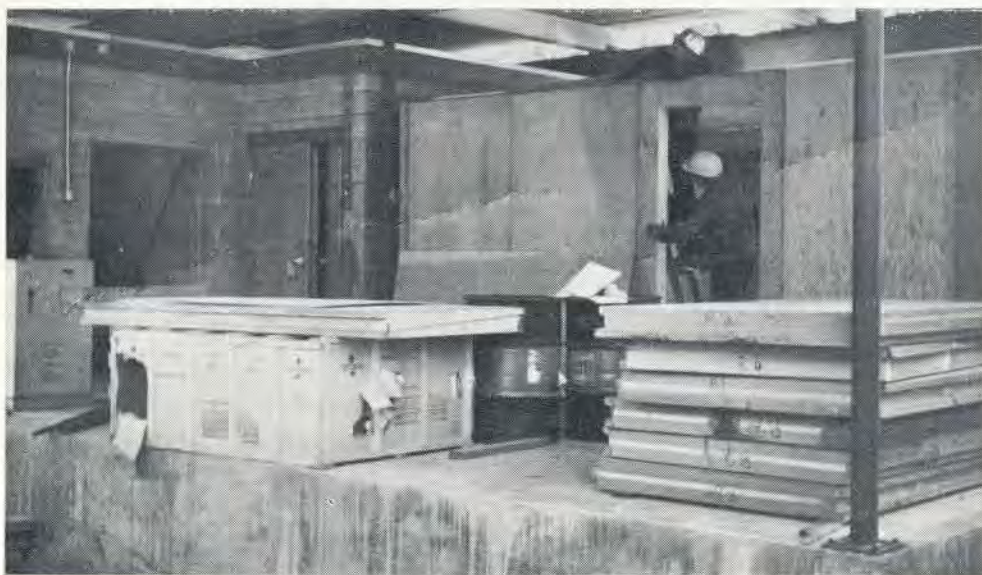
NUMBERED PANELS of plywood and urethane are fitted in place inside of the depot by Konst Construction of Terrace. Some of the numbers can be seen on the panels at the right side of the dock area. The refrigeration equipment was still unpacked at the time this picture was taken.
