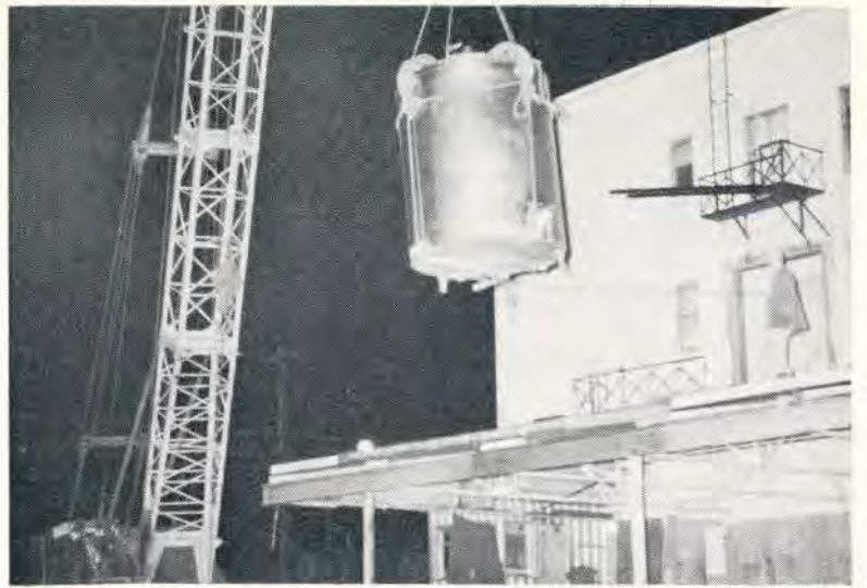
SUSPENDED from a crane behind the Eighth Avenue Plant, this tank is about to be lowered onto a flatdeck truck for transport to the new plant. Much of the moving has been done at night.
