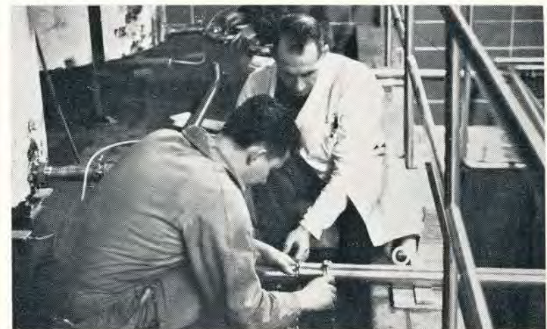
HOOKING UP stainless steel pipe on the processing floor are Doug Wills and Assistant Production Manager Grant Larkin . Fabrication of the pipe system is incomplete.
