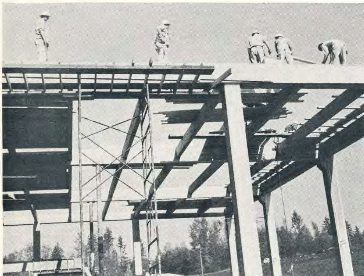
DECKING was being laid on the roof over the powder stores area when this photo was taken a few weeks ago. This section is now finished and roofing
