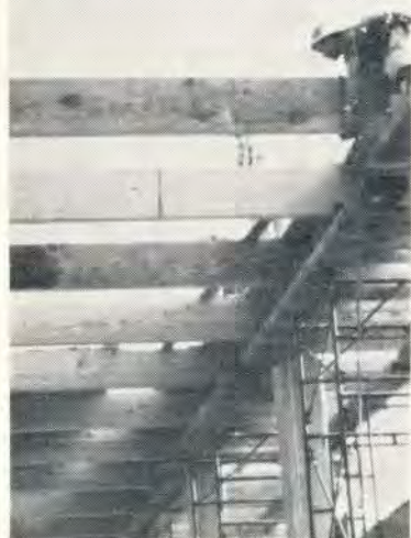
EDGING back to the end of a newly-laid timber, this carpenter has just removed a choker.
