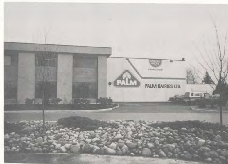
The Annacis facility is thoroughly modern. The plant is about half the size of our Burnaby plant.
