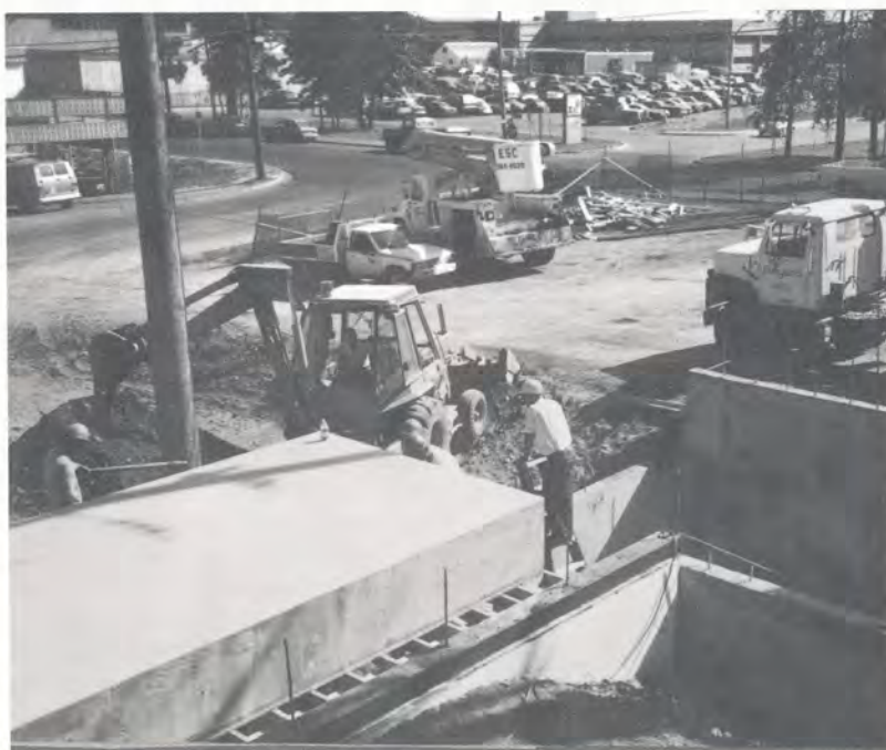
In Prince George, construction employees build foundation for ice builder, which is used during production in the day and to make ice at night.
