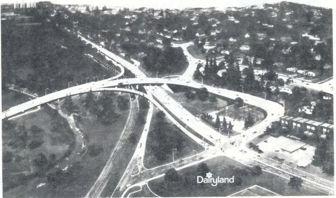
New Railway Overpass Outside Burnaby Plant
