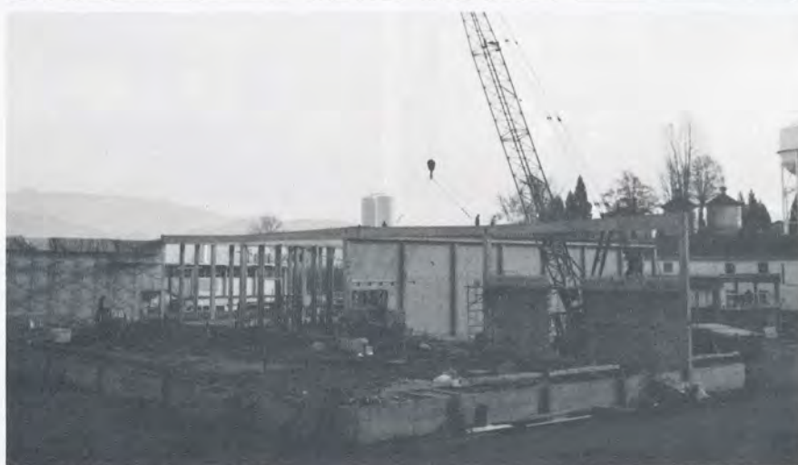
Work is proceeding rapidly on the new Abbotsford plant for future production of Ultra High Temp products and cheese. The roof has been completed since this photo was taken at the end of November. The last of the walls are being erected now and work is beginning on the electrical and plumbing installation.
