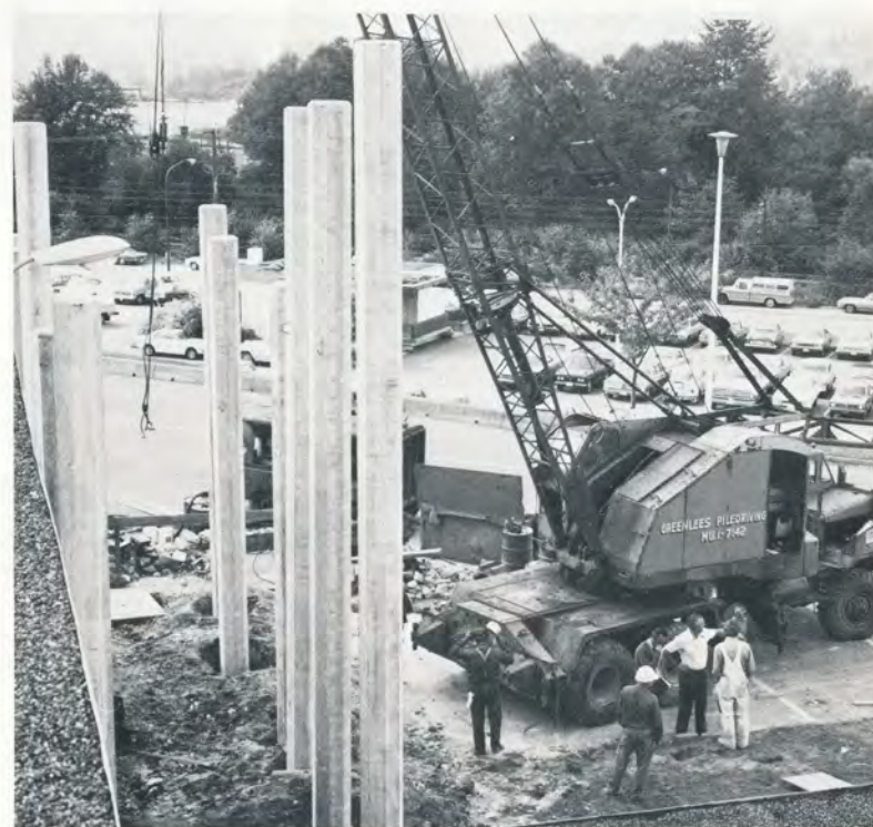
A continual thumping was heard for several days at Burnaby when twelve pre-cast concrete piles were driven outside the plant. They form the basis of support for a four-foot thick concrete platform which is the first step in a planned expansion of the production area. The platform, which will eventually hold three new raw milk tanks, weighs 400,000 pounds and contains 100 yards of concrete. The supporting piles were necessary since the soil in that area contains a three-foot layer of peat which would allow settlement. Holes were first drilled about twenty feet below ground level and the piles were driven down six feet deeper.
