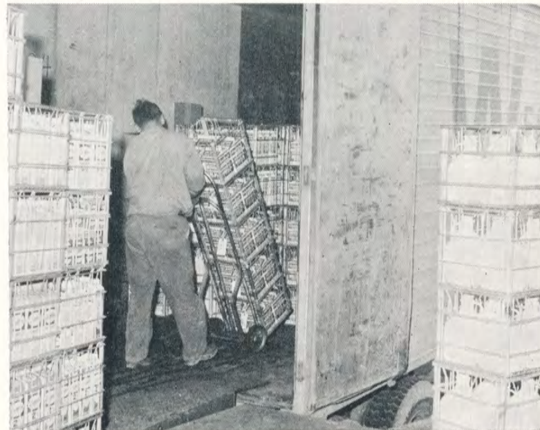
A special feature of the loading docks is the elevating dock boards. By adjusting the dock board, dairy products can be rolled off the dock in to the truck with a minimum of time and effort. Drivers now have to be extra careful when going around the plant because the direction of travel for the tandems is reversed to normal traffic flow.
