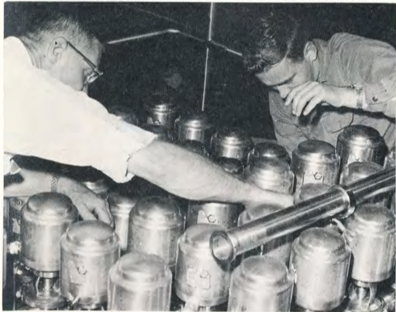
Orie Kroeker, left, and his assistant, worked all night last fall making the changes in the automatic valve system. The valves are located near the holding tanks above the production floor. The valves are made from stainless steel.
