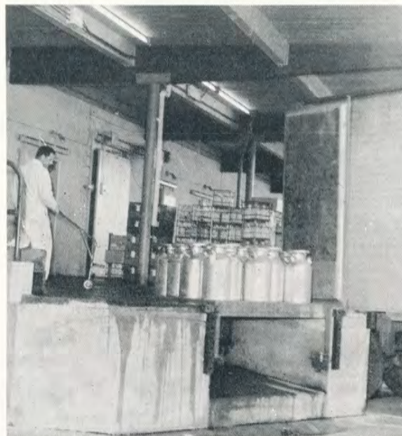
Angle loading docks permit tandem trailer trucks to back in to pick up loads very quickly. Several retail loading bays were eliminated to make way for the new wholesale facilities. The construction was done by Allan and Viner of Vancouver.
