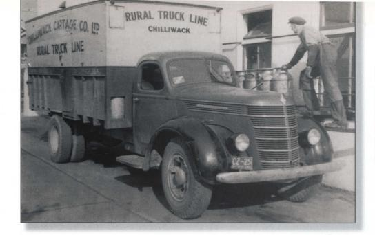
Unloading cans, Chilliwack Cartage, Chilliwack, undated. Chilliwack cartage operated International Harvester single and tandem-drive trucks. All were covered vans, affording the milk some protection from the weather.
